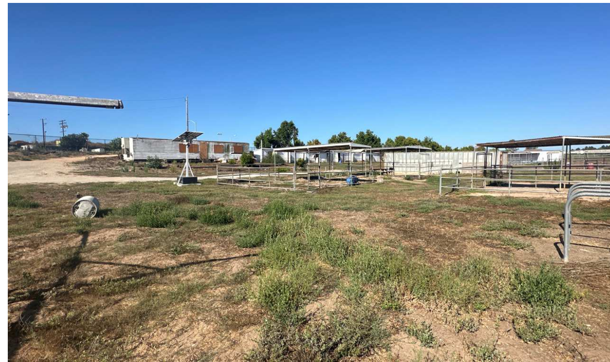
Photograph 4: View looking southwest at the remaining equestrian infrastructure (August 21, 2024).
