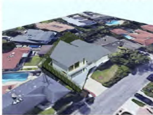
AERIAL VIEW - SOUTHWEST STREET FRONTAGE
